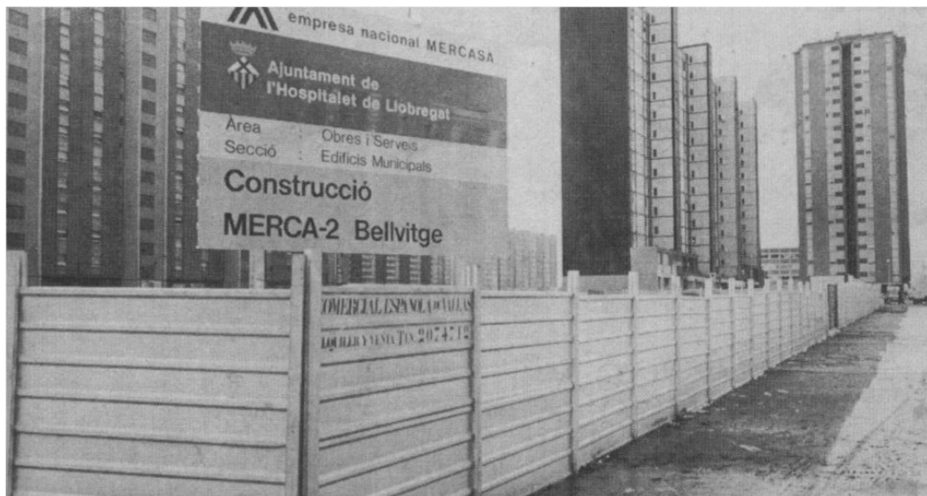
Pic 3: The construction of Bellvitge
